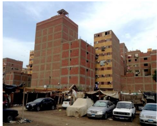
Figure ( 5 )Cairo's Red Brick Neighborhoods
